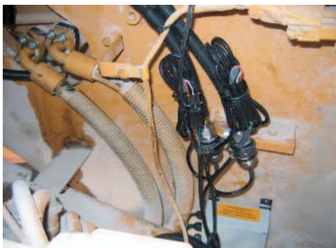
Cat Load sensor installation
